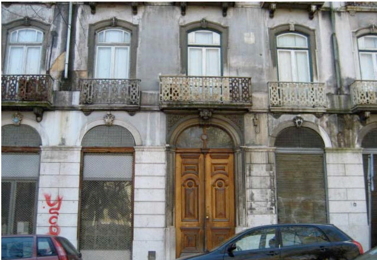
The main gate of the Avenida Liberdade 195 – 211 in Lisbon
